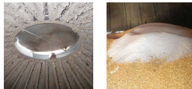
5. Moisture below dripping down spouts or vents from snow or rain:
