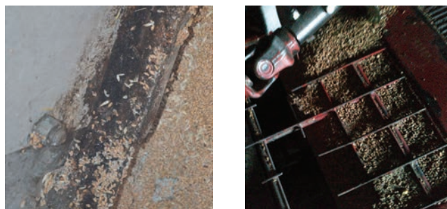
2. Crusted grain hang-ups and clumps from missing bolts or grain debris left on the floor and augers:
