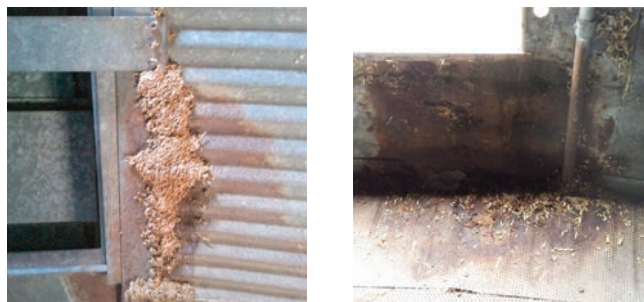
3. Grain clumps on side doors or on the holes of the bin walls:
